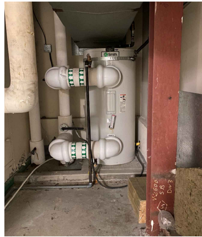
F EXISTING BUFFER TANK M2.202 SCALE: N/A
