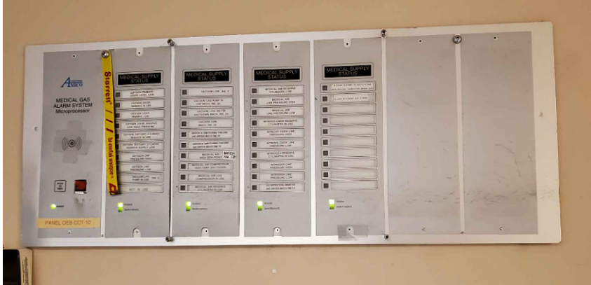
C MASTER ALARM PANEL IN SWITCHBOARD M2.104 SCALE: N/A
