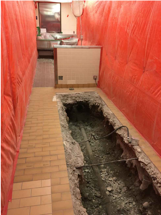
24 M501 PREVIOUS PHOTO OF EXCAVATION FOR SANITARY PIPING REVISIONS (FOR INFO ONLY) NTS
