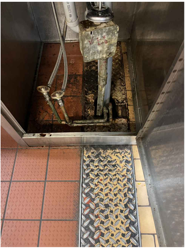
6 M500 EXISTING TRENCH DRAIN NTS
