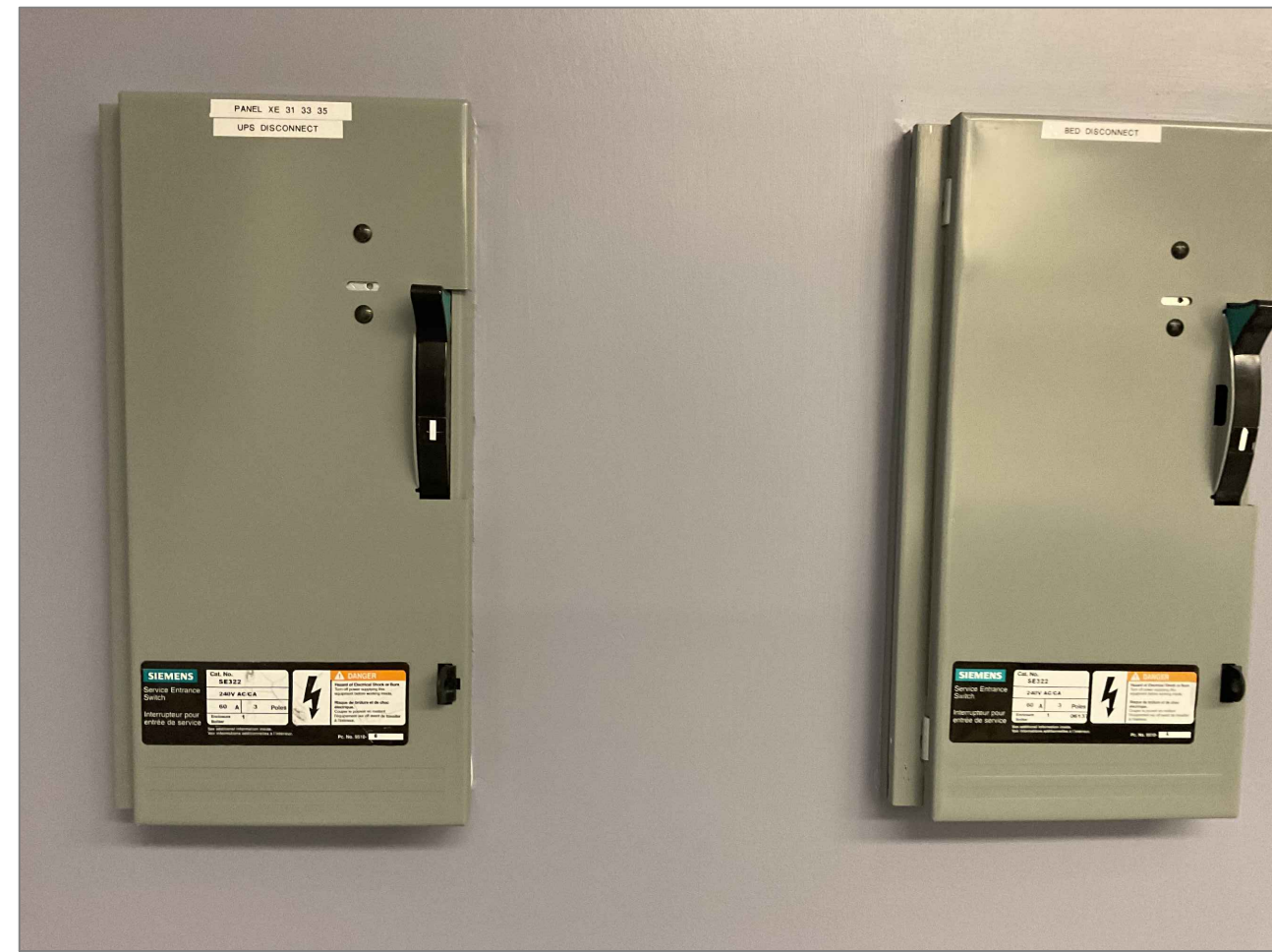
4 UPS DISCONNECT SWITCH IN THE SCAN ROOM TO BE REMOVED SCALE: 1:30
