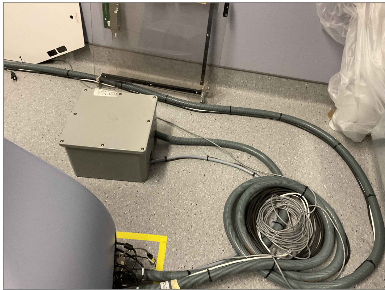
3 JUNCTION BOX IN THE SCAN ROOM TO BE REMOVED BACK TO THE SOURCE SCALE: 1:30
